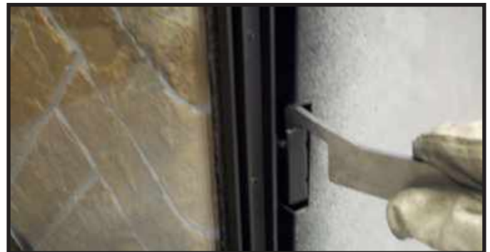
Figure 11.7. Securing Side Glass Clips
