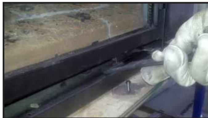
Figure 11.2. Glass Clip Tool Location
