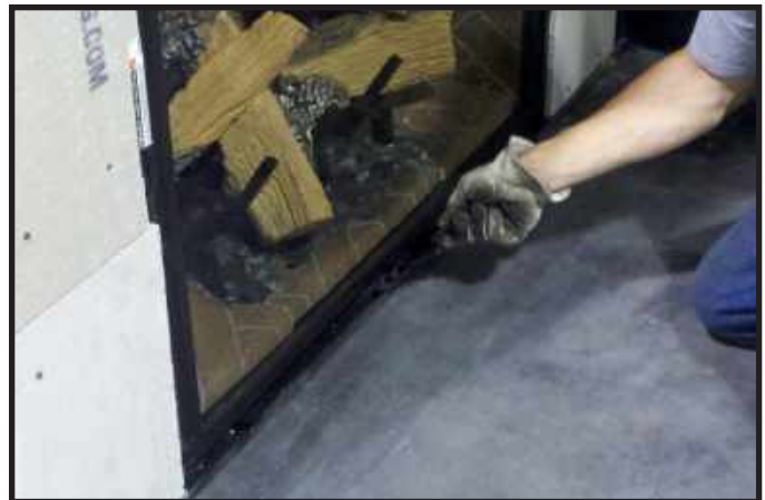
Figure 11.8. Securing Bottom Glass Clips
