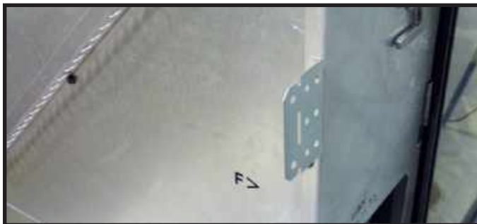
Figure 6.4 Nailing Tab Bent Out for Installation
