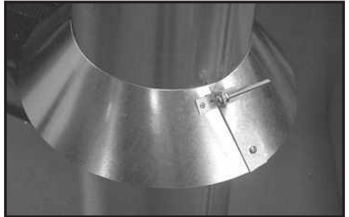
Figure 7.12 Insert Bolt into Brackets
