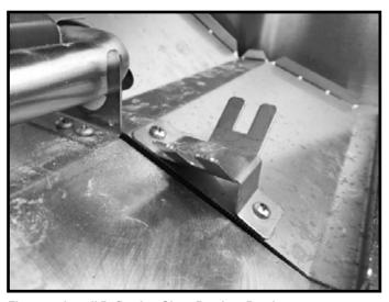
Figure 5. Install Deflection Glass Retainer Brackets Outdoor Lifestyles by Hearth & Home Technologies • Courtyard Contemporary Hearth Kit • 4608-906 • 3/18
