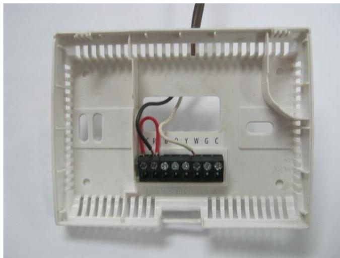
Connect one wire on “RH” and the other wire on “W”. Red wire jumper can remain installed. For further information refer to the manufacturer's instructions.
