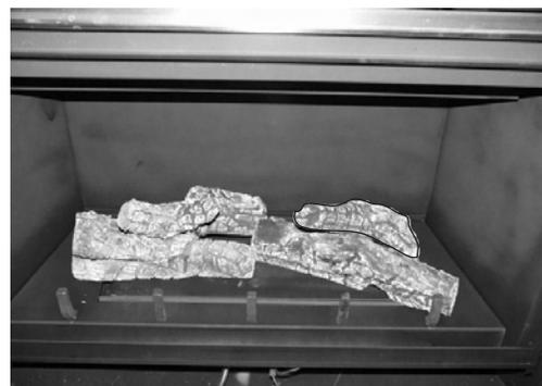
**STEP 7** - Locate Log #4 locator tab in the back right hand side of firebox. Butt Log #4 up to locator tab. Position short Y branch onto ledge (rear section) of Log #2. NOTE : Ensure at this time that logs are not sitting directly on top of open gas ports.
