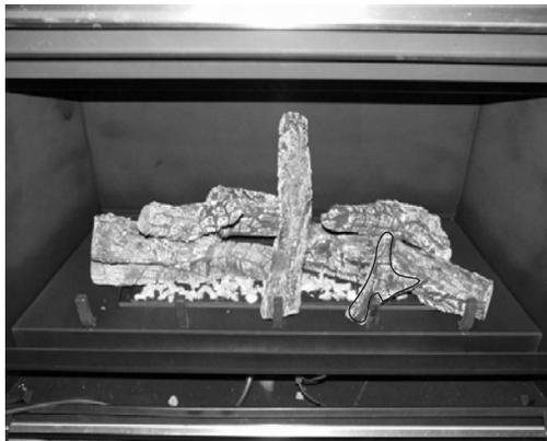
**STEP 10** - Position Log #6 up against the 2nd grate from the right. Log #6 will rest onto Log #2 (Do not position over main burner ports).
