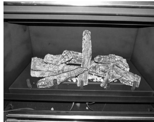
**STEP 11** - Lean Log #7 against the 2nd grate from the left and notch on Log #5 (Do not position over burner ports).
