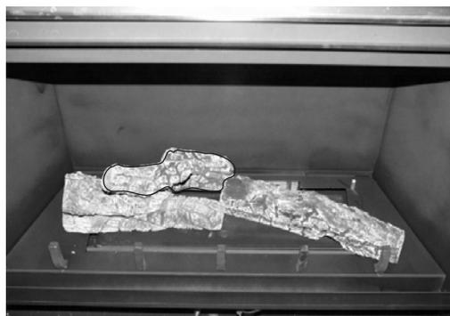
**STEP 6** - Locate the log locator tabs for Log #3. The notched area of Log #3 is to be positioned up against the two tabs and rests onto Log #1 (as illustrated).
