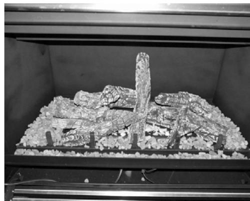
**STEP 12** - Place rock onto the false bottom only. NOTE: Do not cover air slot that is between grate and false bottom.
