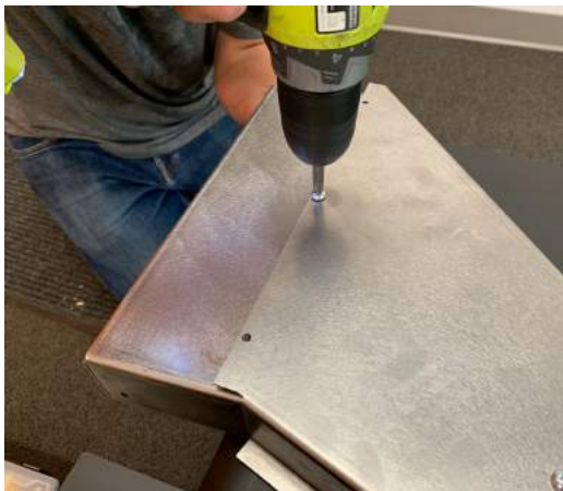
Attach top rear blower duct to top middle blower duct piece
