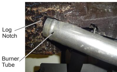
**Figure 25A - Installing Back Left Log**
