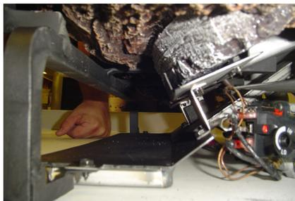
**Figure 24C - Installing Right Front Log, Side View**
